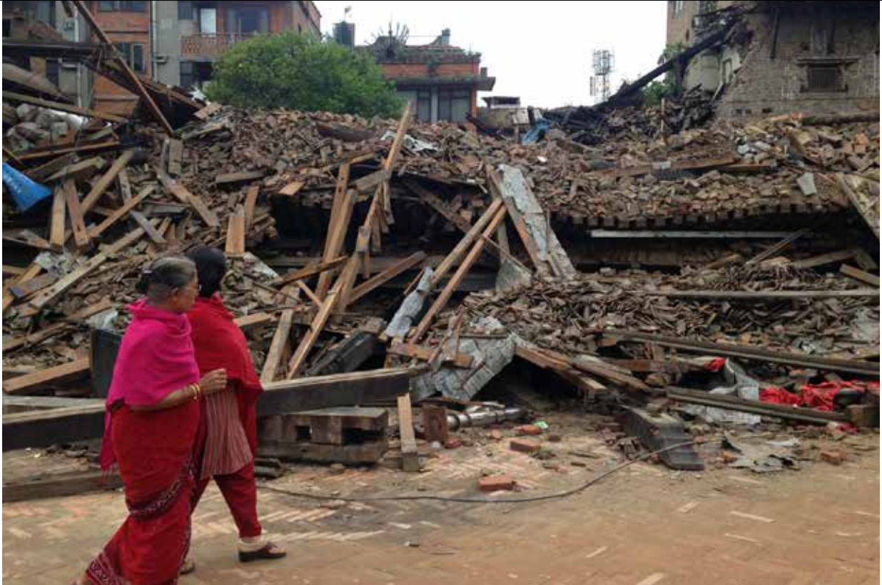
Earthquake destruction, Bhaktapur
